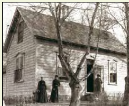
Niels Johnsons hus.
