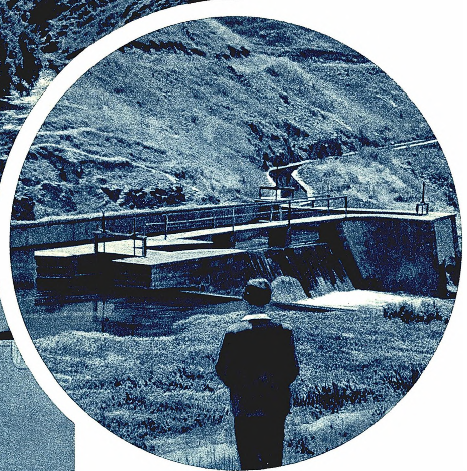
A power dam, curbing a turbulent mountain stream.
