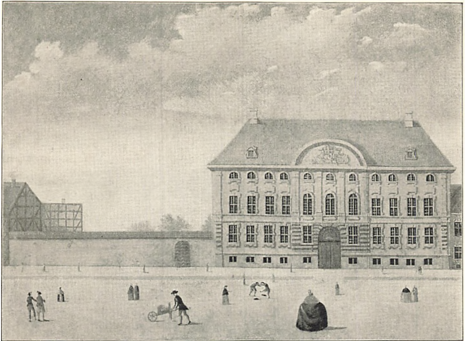
GREV DANNESKIOLD-LAURWIGENS PALÆ, STORE KONGENSGADE 68.
