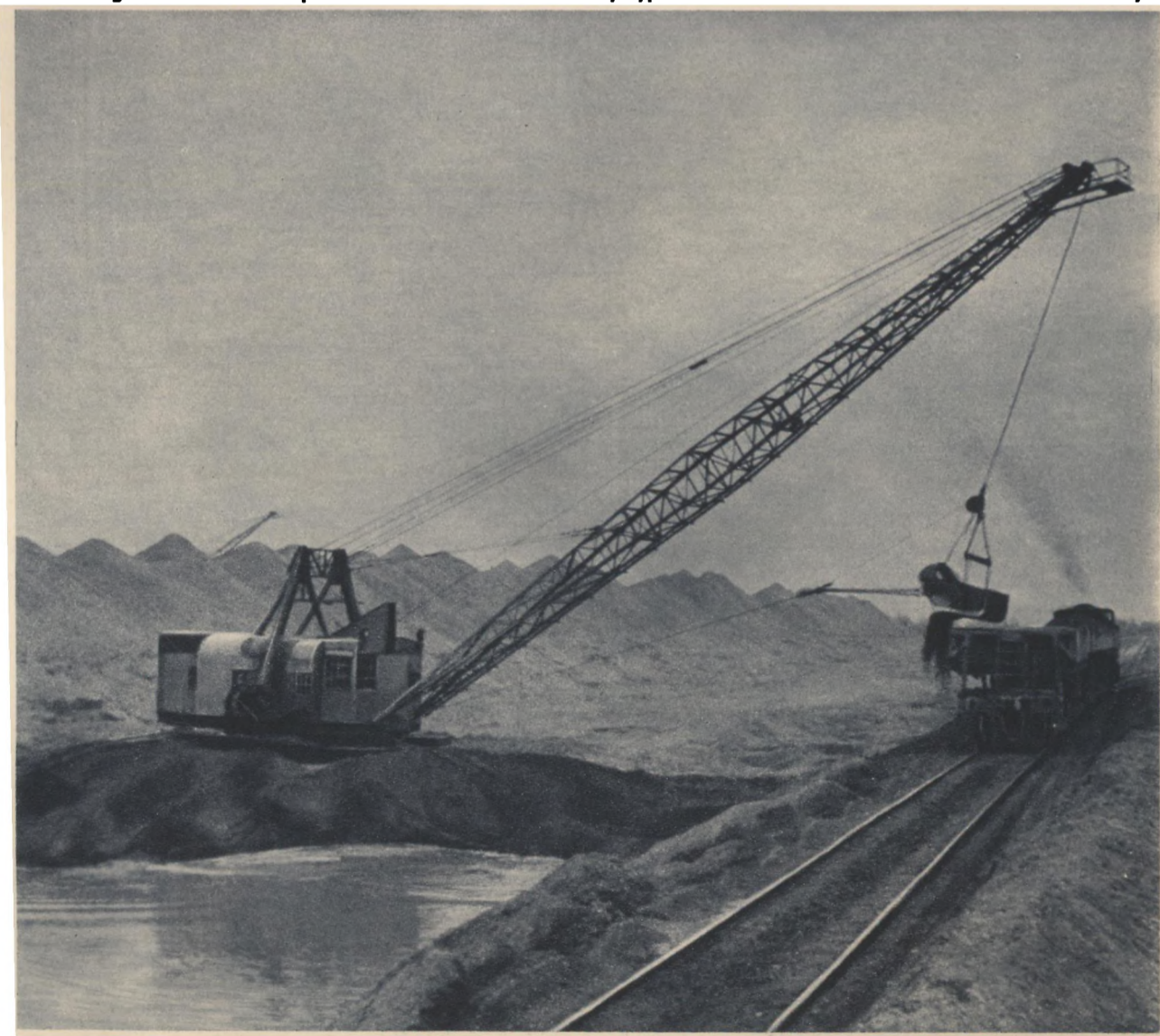
The walking excavator in the photo below is one of the many types of modern Soviet-made machines used on the job
