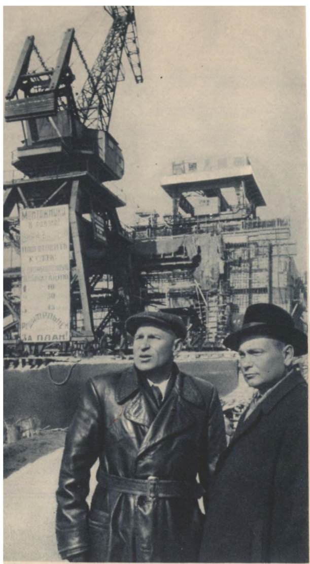
Engineers Pavel Shelukhin and Andrei Popov who with a group of other workers on the Tsimlyanskaya Power Plant were awarded a Stalin Prize for accelerating the building of the earth dam by a hydraulic process
