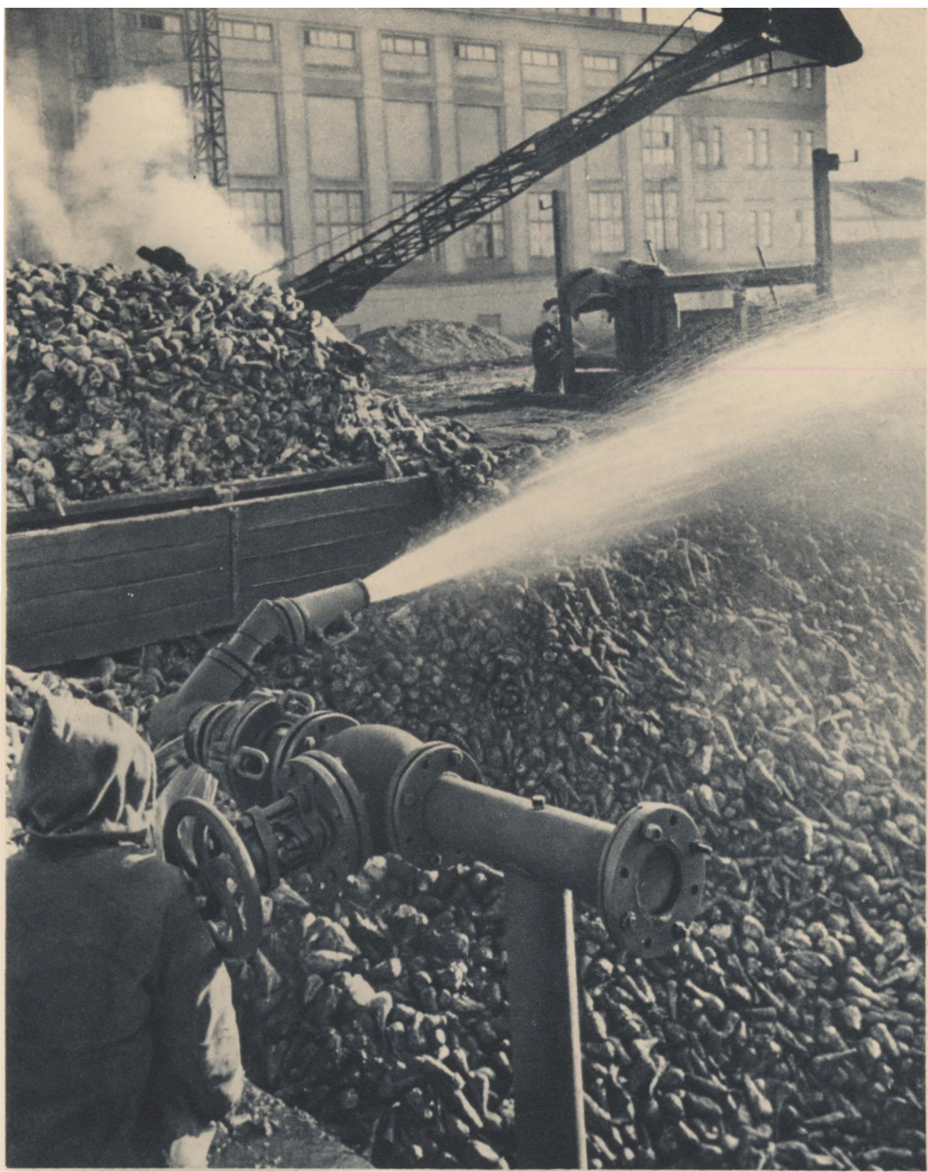
Trainload after trainload of sugar beet is delivered to the refinery, where it is unloaded by machines and transferred to the washing department by monitons
