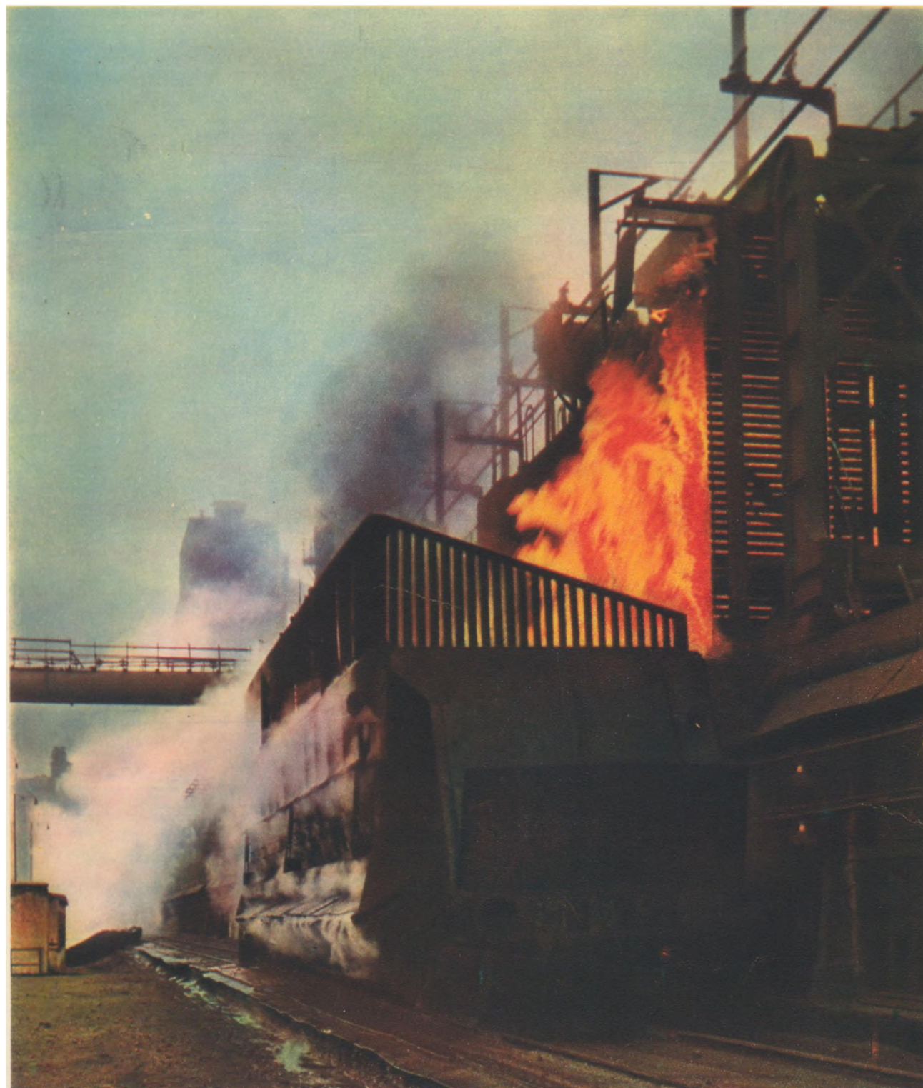
One man at a switchboard operates the coke-discharging machine which removes the doors of the coke ovens, extracts the coke, puts the doors back in place and levels the charge
