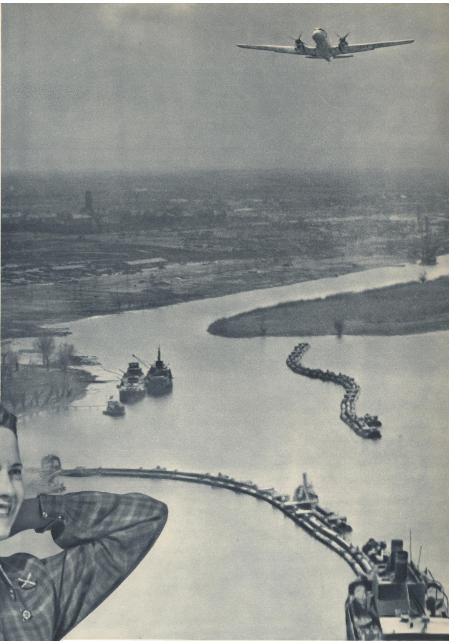
The Dnieper River at the city of Novaya Kakhovka. The foreground shows a suction dredge at work at the hydroelectric development site
