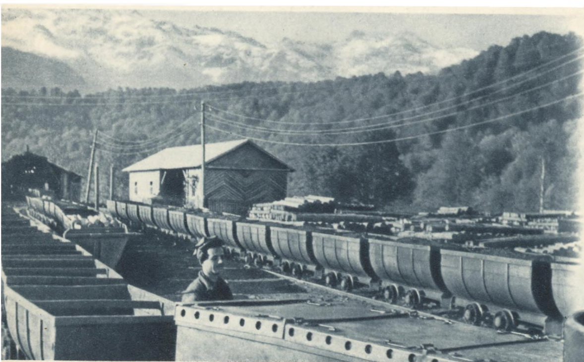
Near one of Tkvarcheli mines. Electric locomotives hauling train-loads of coal reach the surface
