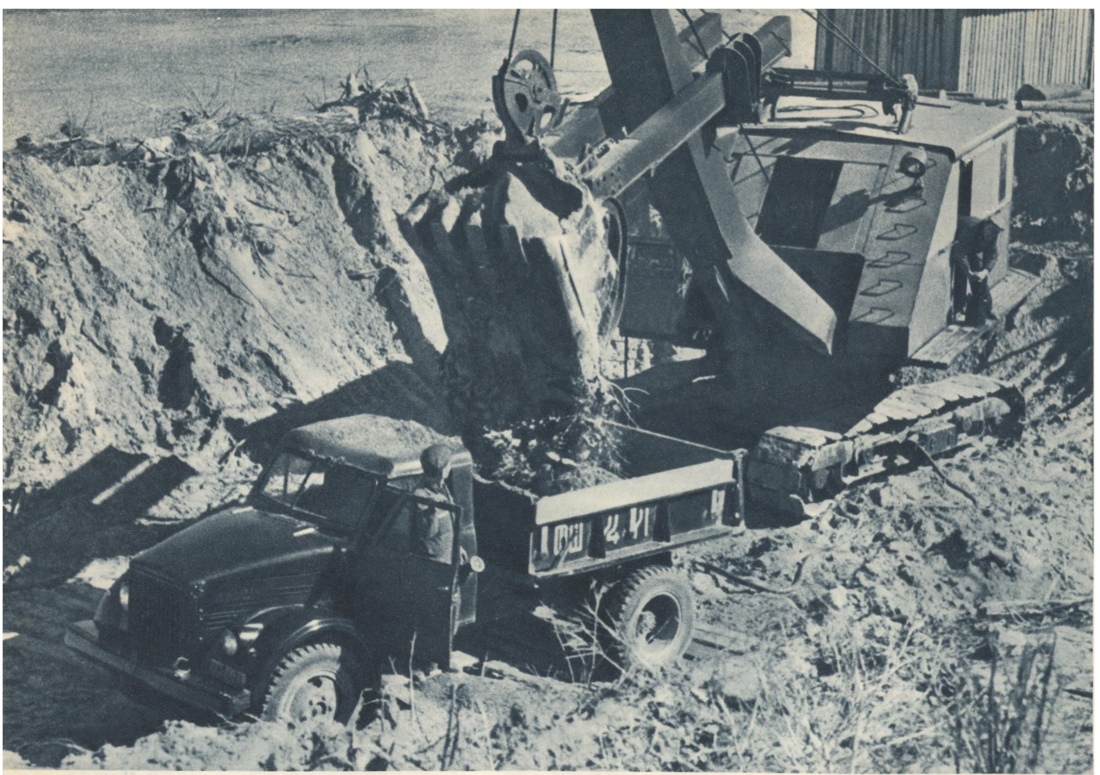
An excavator in action on the foundations of the Kakhovka dam
