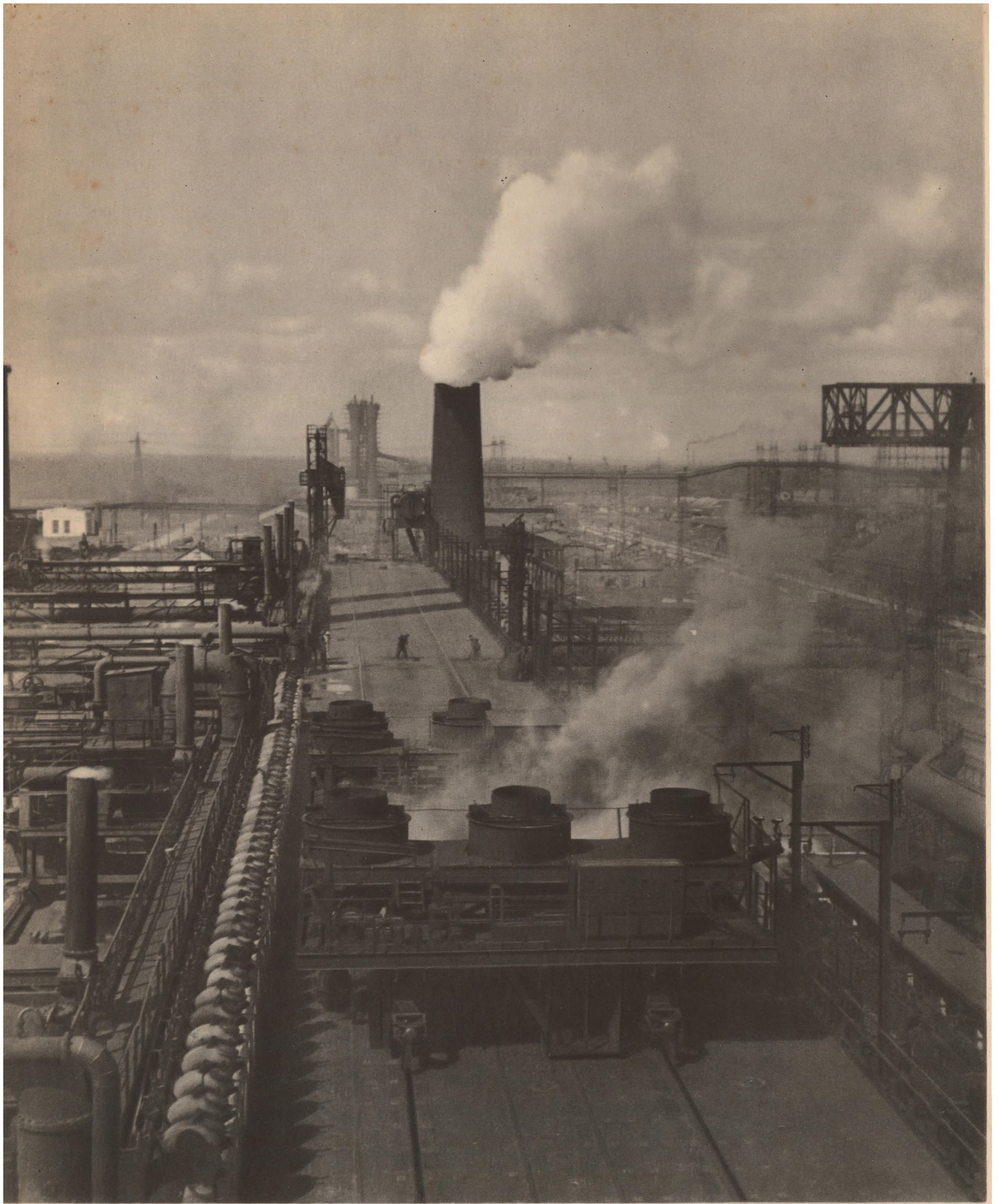
Coke oven batteries at the Zaporozhye Coking Plant (see "Reply to a Swiss Reader" on pp. 10-13 of this issue)
