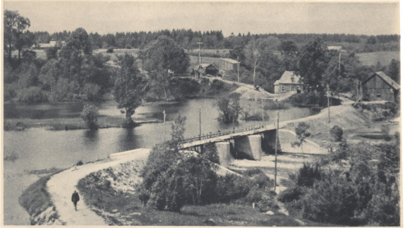
A rural hydropower station on the river Virvite, in Kursenai District, Siauliai Region. It supplies five collective farms with current
