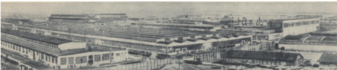
General view of the first Soviet tractor factory, built in Stalingrad, as it looked in 1933
