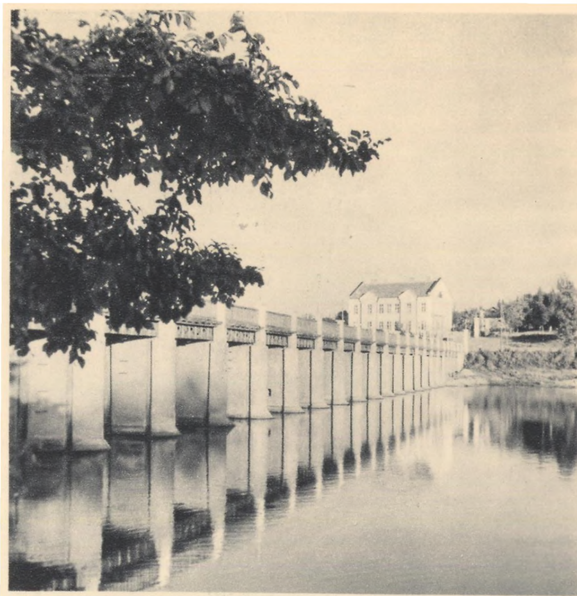
View of the Korsun-Shevchenkovsky hydroelectric station in the Ukraine which serves many collective farms in the district. Below: Ploughing by electric tractor at one of these collective farms. The electrification of Soviet agriculture is being considerably expanded
