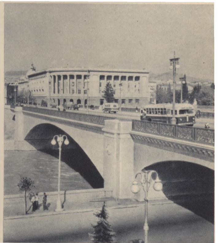
TBILISI. This new bridge across the Kura is one of the features of the big municipal construction programme in the capital of Soviet Georgia Photo by G. Kvirkuelia
