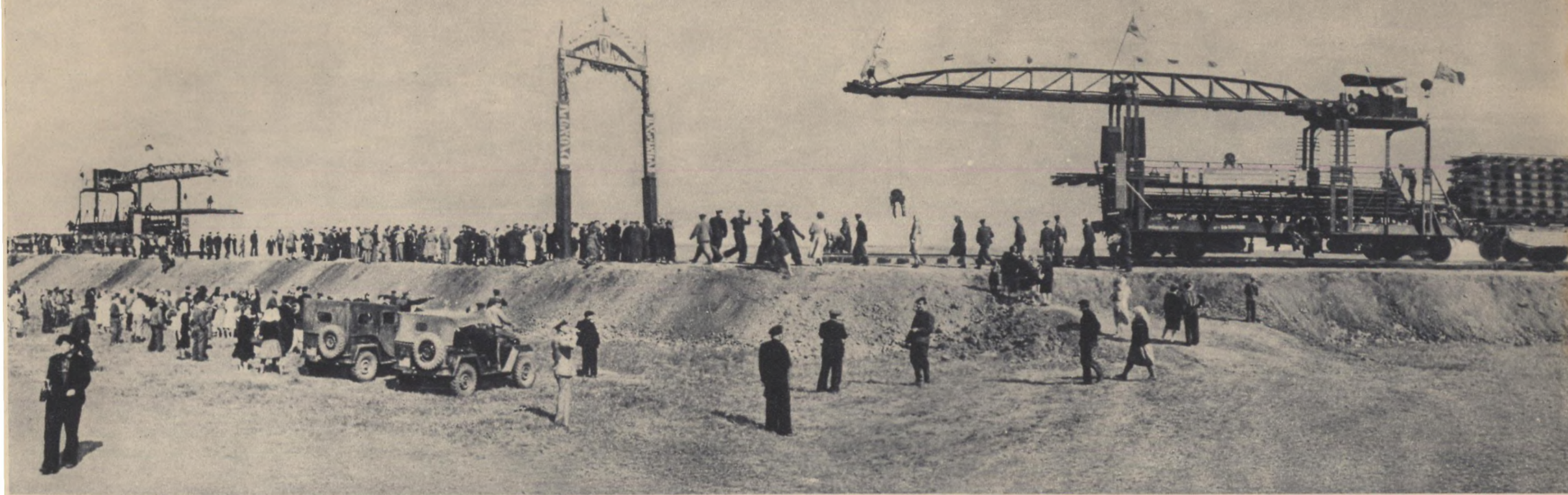
KULUNDA. These track-laying machines are putting down the last yards of the Barnaul-Kulunda section of the South-Siberian Railway. The section was completed on May 24, not long after the Stalinsk-Barnaul section was commissioned. A tracklayer does the work of 700 labourers. Upwards of 4,000,000 cubic metres (141,200,000 cubic feet) of earth was excavated at the construction job in a short period of time; 15,000 cubic metres (529,500 cubic feet) of concrete and ferro-concrete was placed, and 350 kilometres (about 220 miles) of main and station tracks laid. Stations and workers' settlements with clubs, shops, schools, and hospitals have been built on the section
