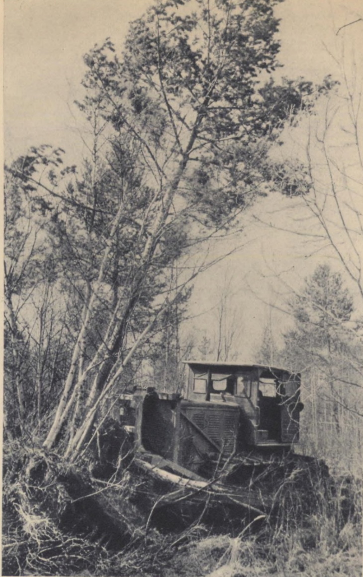
LATVA. Stubbing and gathering machines blaze trails for reclamation machinery in the marshes of Prionezhsky District, in the Karelo-Finnish Soviet Republic. Reclamation stations in the Republic are draining and clearing bogs on a large scale Photo by P. Bezzubenko
