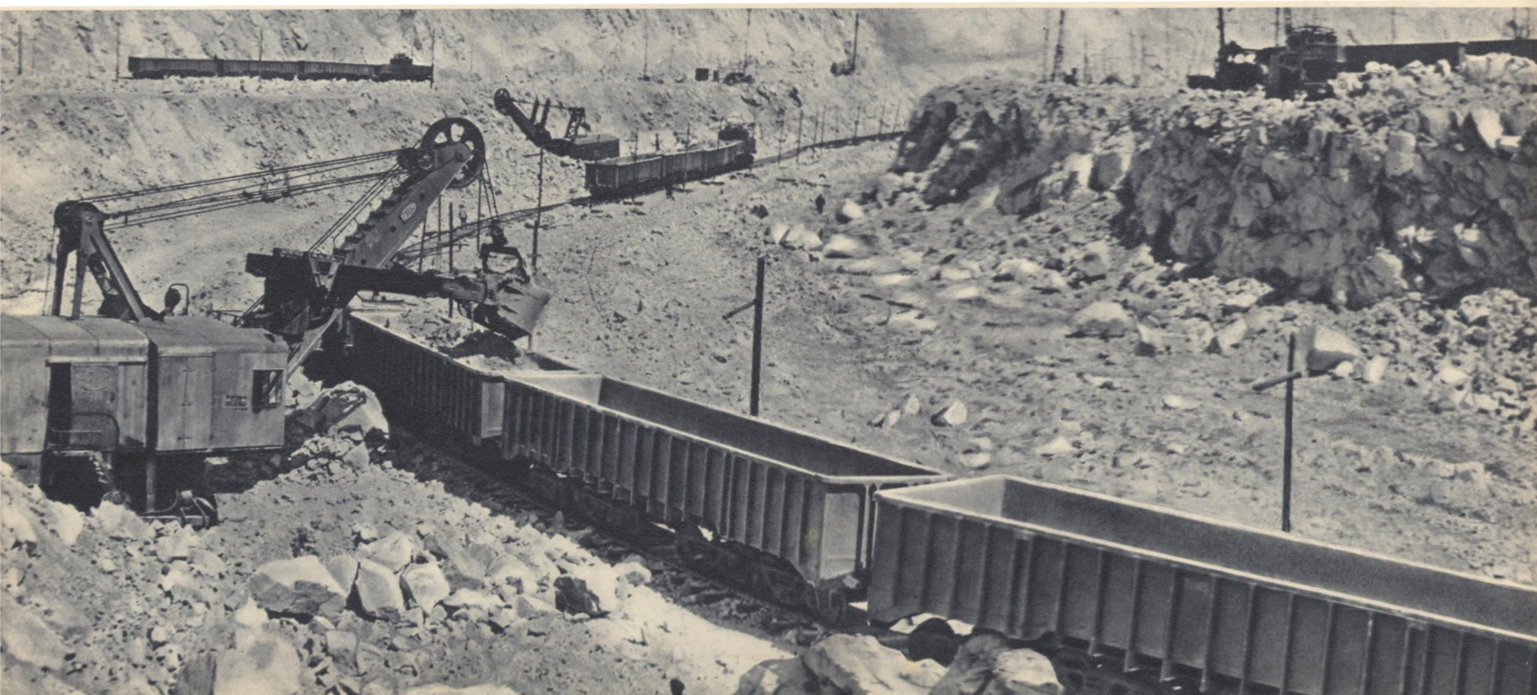
Loading copper ore into gondola cars at the Kounrad mine
