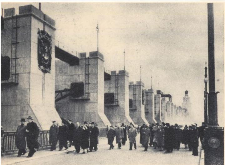
Inspecting the dam of the Tsimlyanskaya Hydroelectric Station
