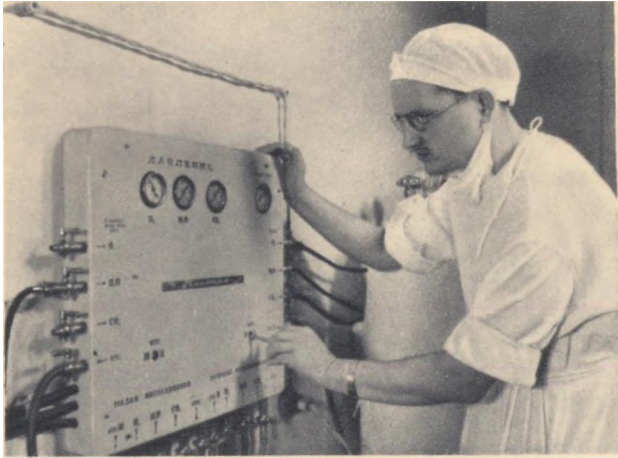
At the control panel in the apparatus room adjoining the operating theatre, S. V. Ryneisky prepares a gas anaesthetic
