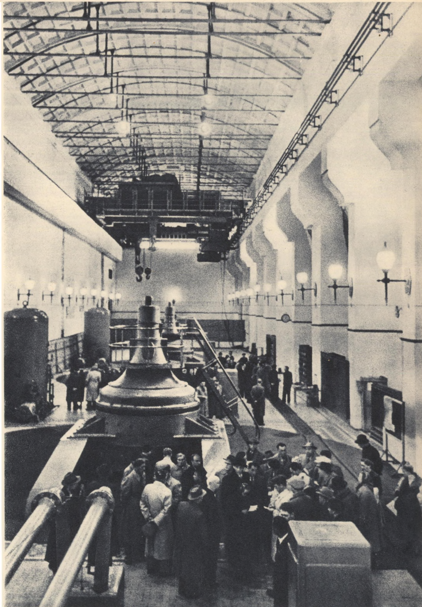
The visitors from abroad displayed great interest in the turbine hall of the Tsimlyanskaya Hydroelectric Station
