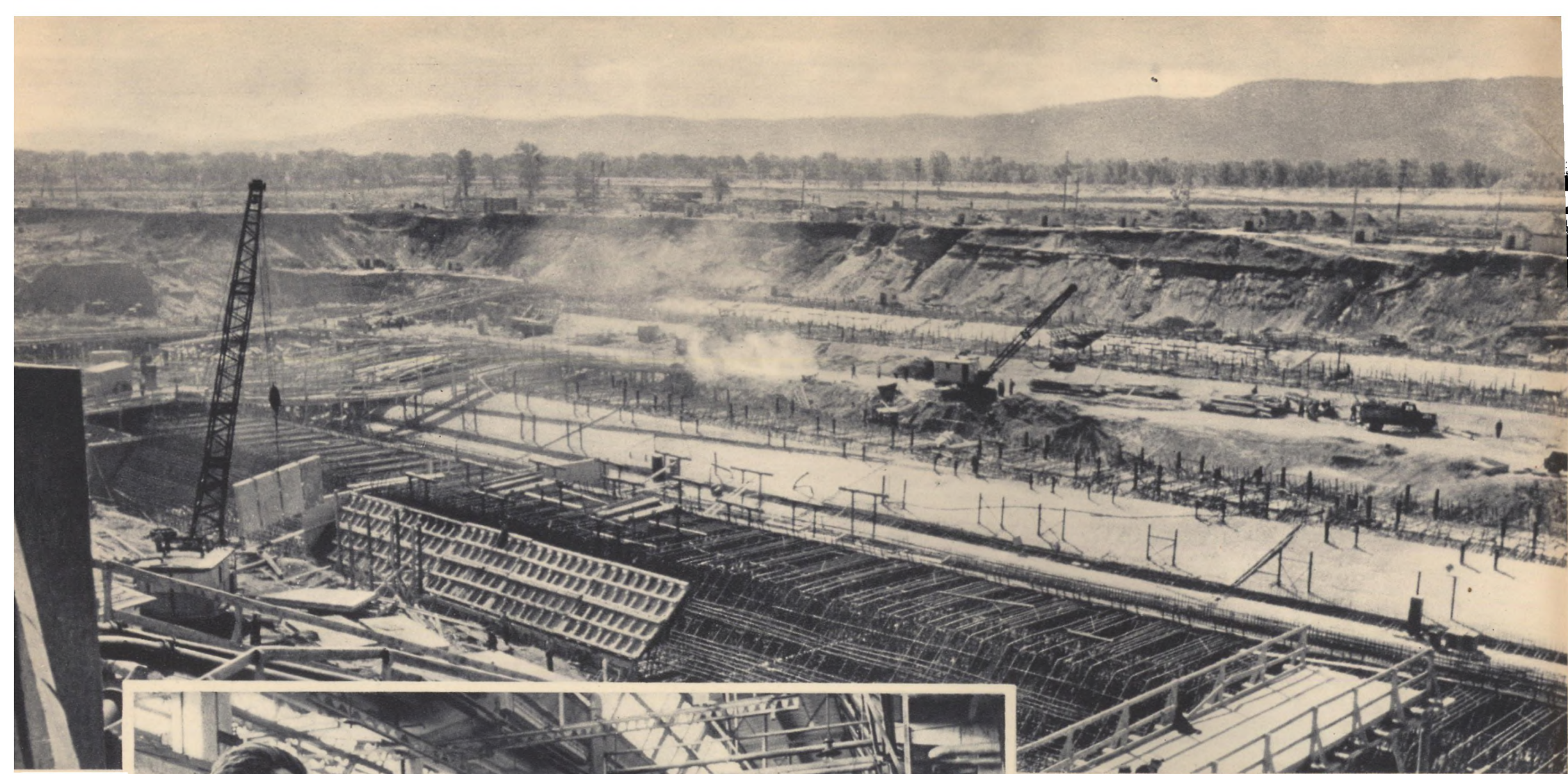
KUIBYSHEV. A general view of the construction pit of the lower shipping lock of the Kuibyshev Hydroelectric Station. The builders pledged to fulfil their eight months' quota by August 21, the third anniversary of the Government's decision to build the power station, and they are making good their word
