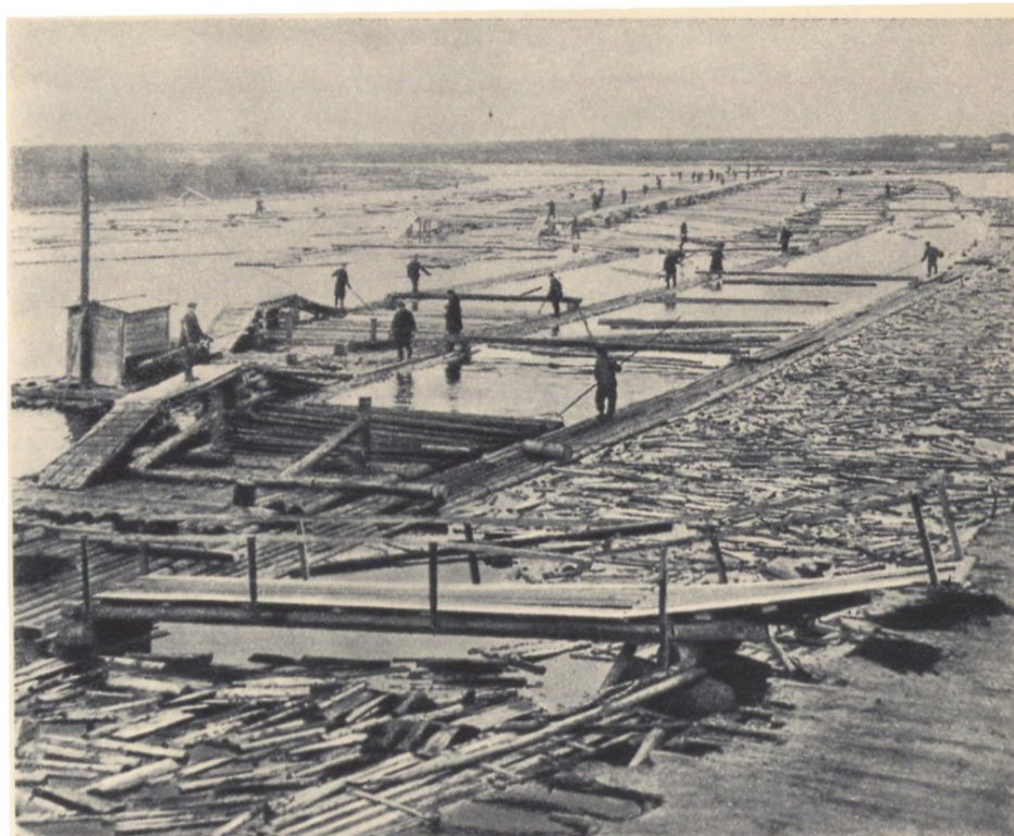
Timber sorting on the Oyat. After skilled rafterers have sorted the timber the logs are bound by machines into sections which are combined later into rafts
