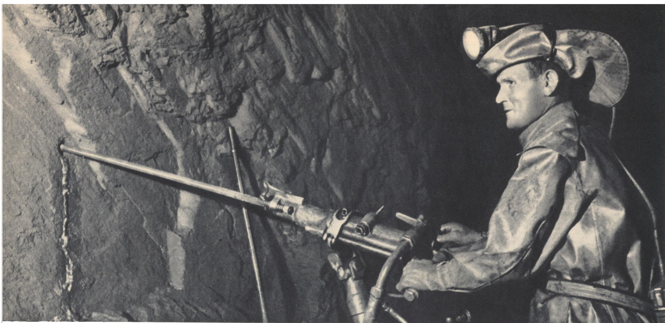
Wet boring is employed in many coal and ore mines to combat dust. Water is piped to the face and hoses are attached to the perforating picks. Here V. Urbalevich, a tunneler, is seen using this method in the Novaya Pit at the Dzerzhinsky ore field Photographed by S. Viltman
