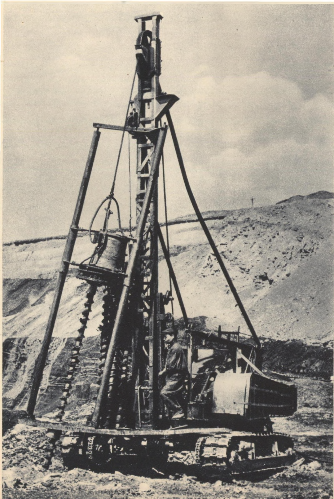
Left: A frame for drilling the coal seam obliquely
