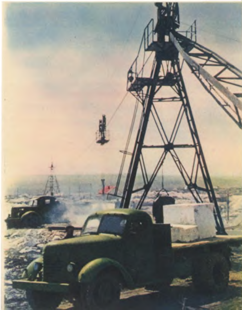
Below: Loading marble extracted from the Koelga Quarry
