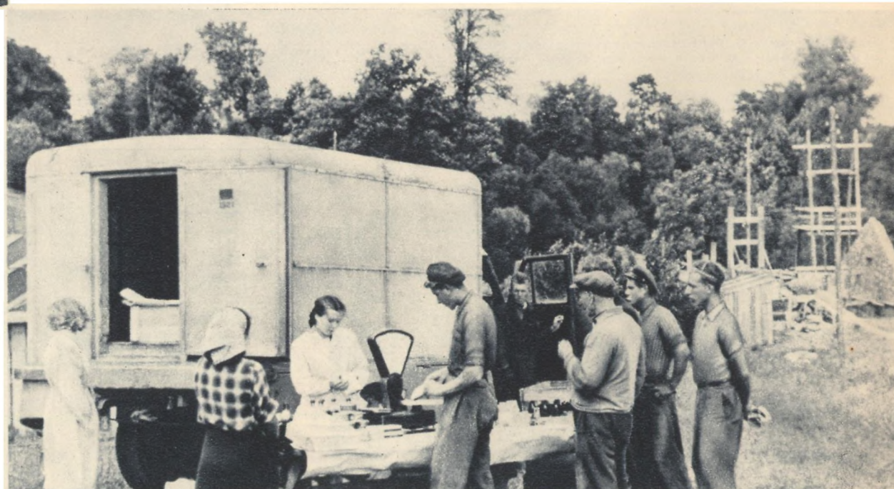
One of the shop's mobile stalls does a brisk trade at the construction site of an inter-kolkhoz power station
