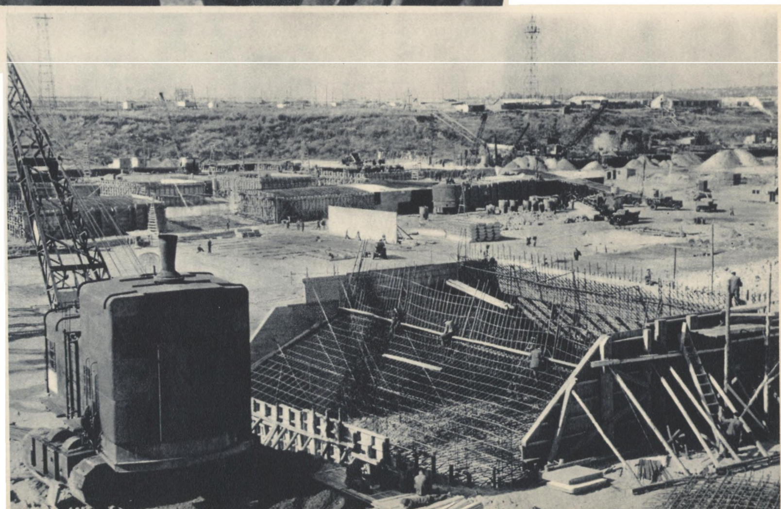
Building an abutment for the power-house
