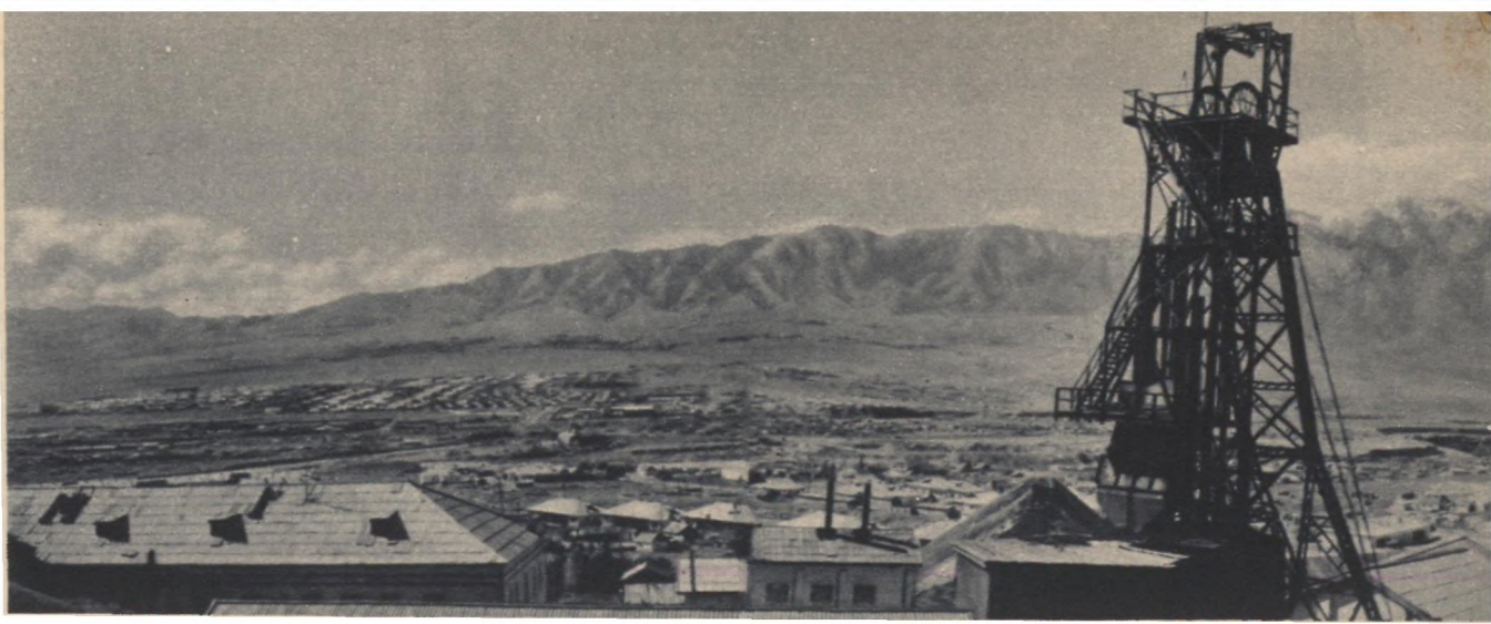
Headframe of Pit No. 9. Angren coal is mined deep underground as well as by the open-cut method
