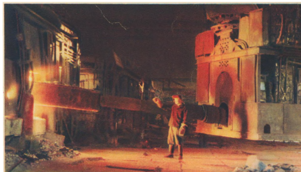
Charging an open-hearth furnace with a loading machine
