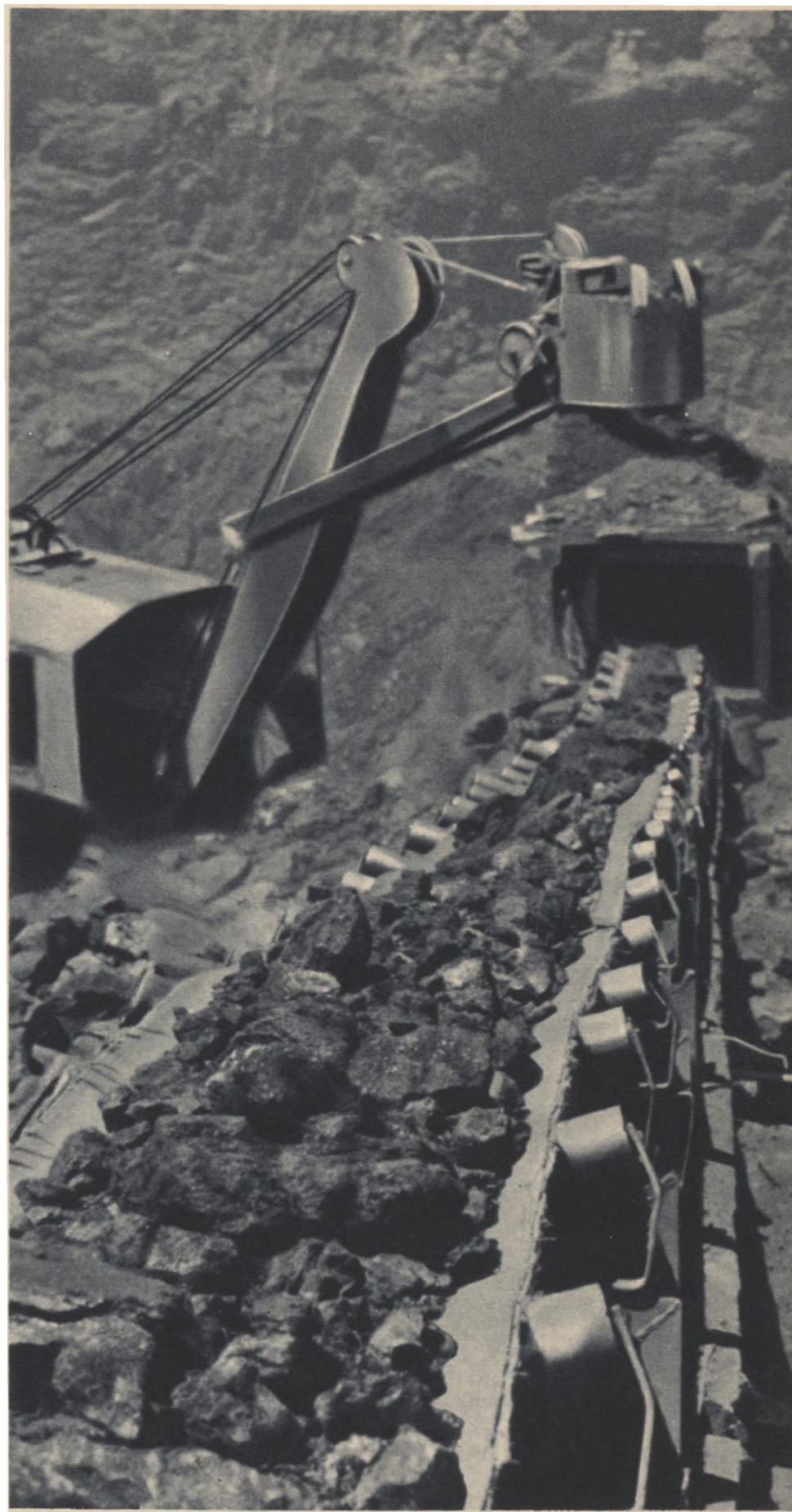
Coal removed from the open-cut working by power excavators flows along conveyor belts in a steady stream
