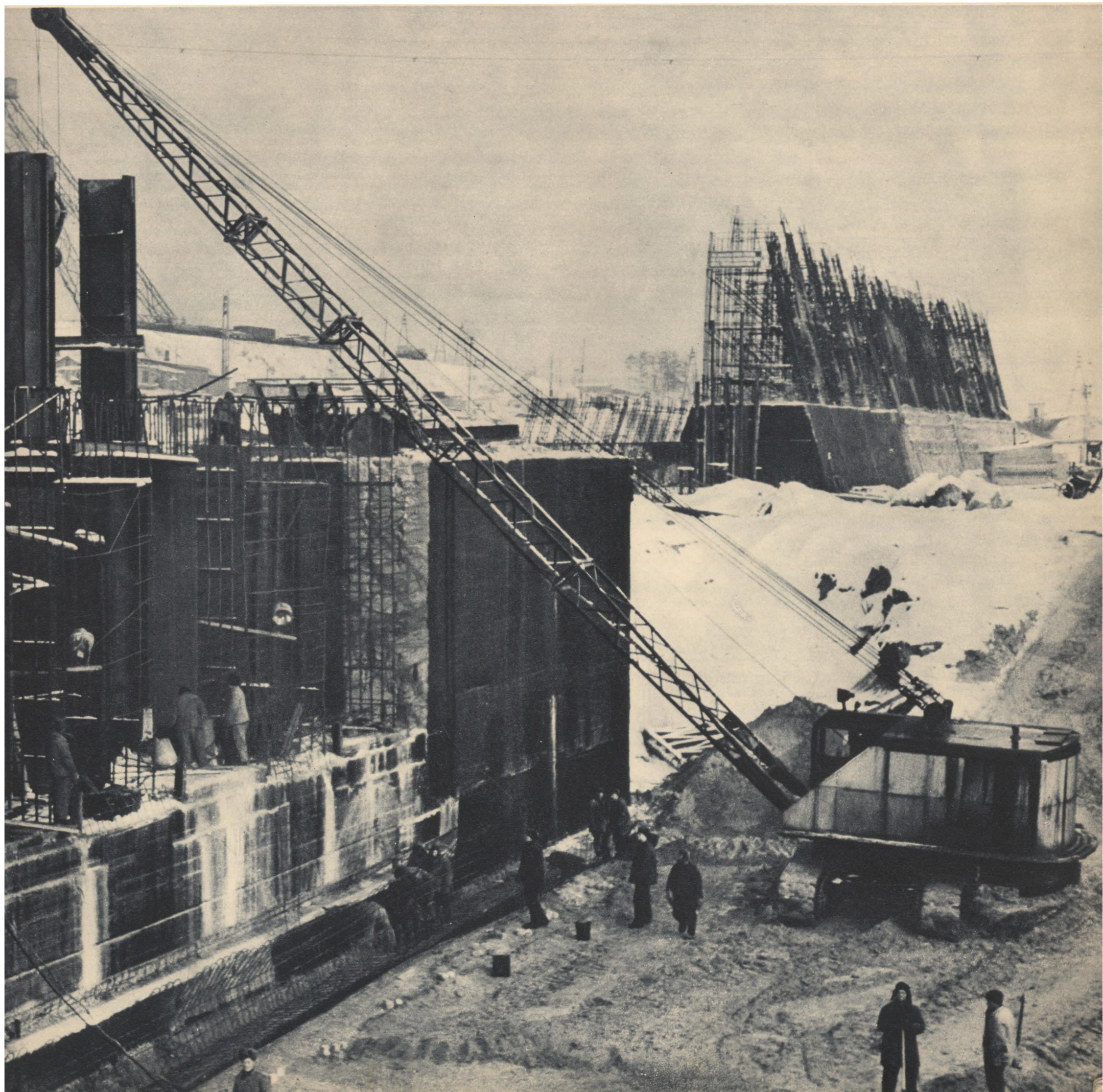
The elevated concrete-discharge track (above) and the lower navigation lock (below) under construction
