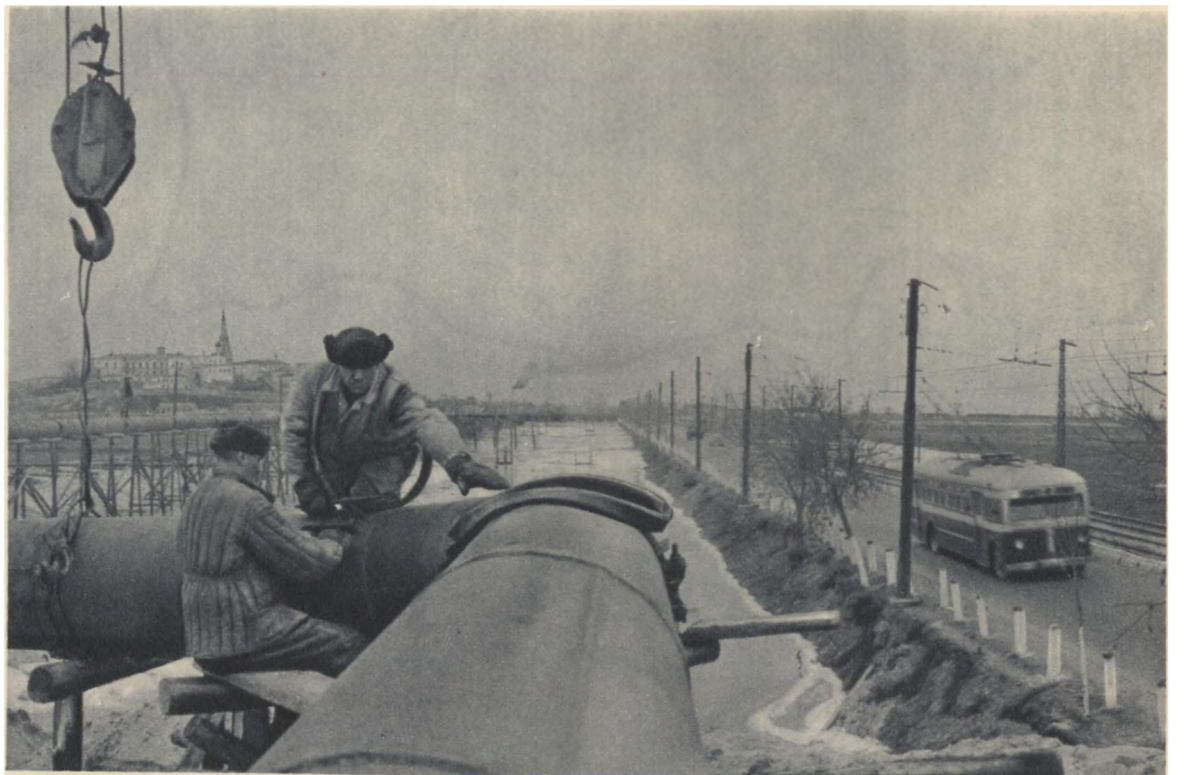
Gabbas Habibullin's crew is assembling a pipe line that will carry soil from suction dredges to build up a dike
