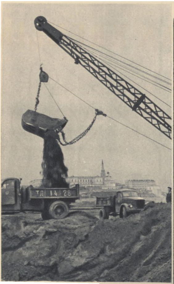
Mechanical shovels remove millions of cubic feet of earth from the construction area
