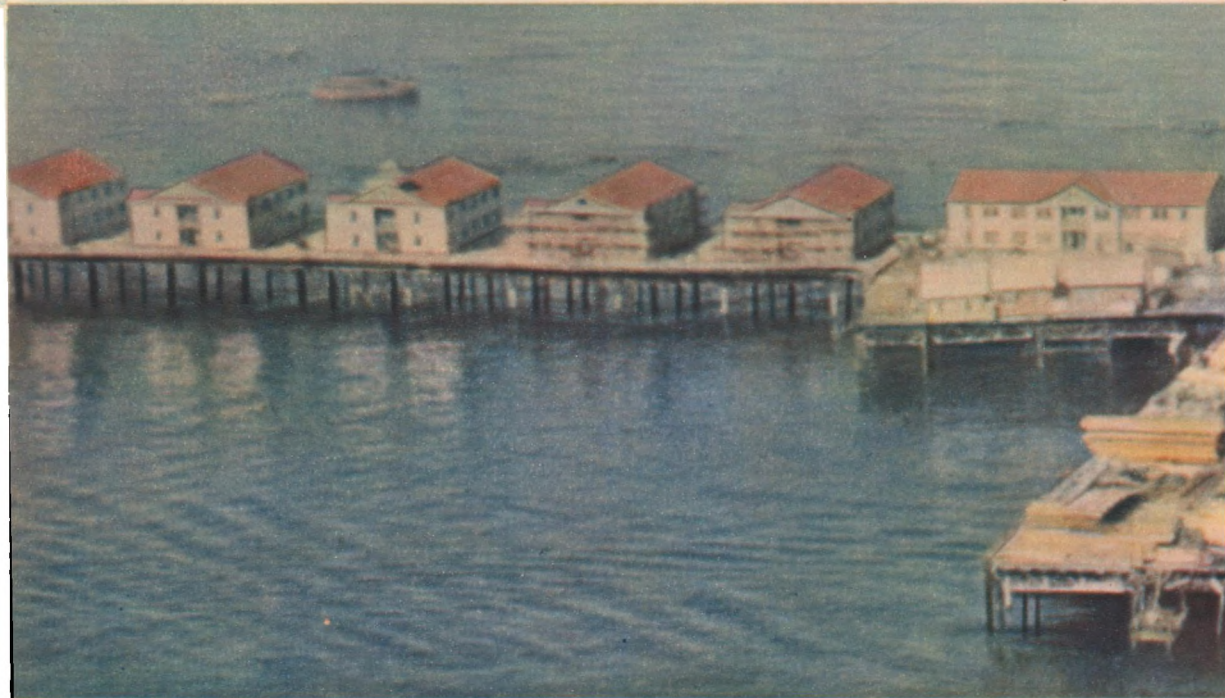
Right: A section of the oil workers' town that has been built on steel piles in the Caspian →
