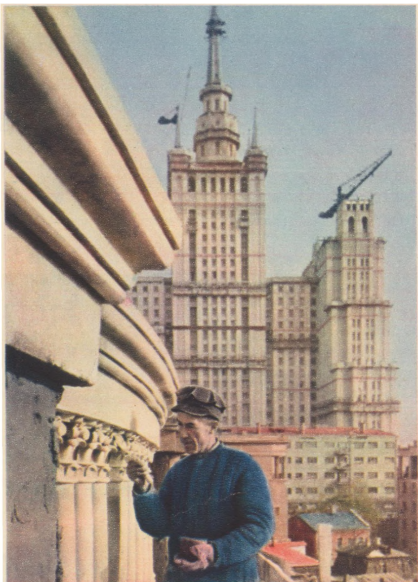
Work on the outside of Krasnaya Presnya Station is in its final stage
