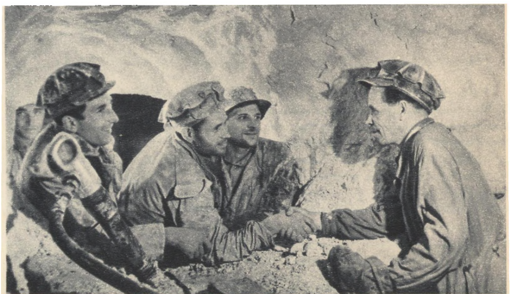
A memorable moment in the construction of the last section of the Main Belt. Two brigades of tunnellers, working from opposite ends, meet underground
