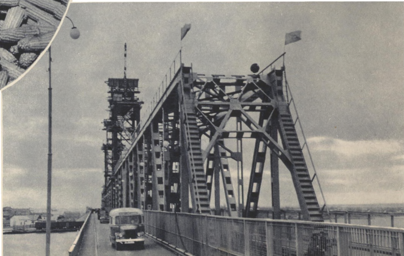
UKRAINIAN REPUBLIC. Dniester Bay Bridge was opened for traffic a fortnight ahead of schedule Photographed by A. Fateyev
