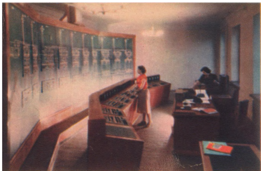
← The central control room of the Leningrad Metro
