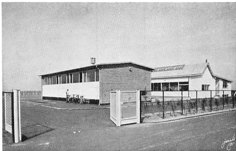
Kloakpumpestationen i Skovshoved 1941.
