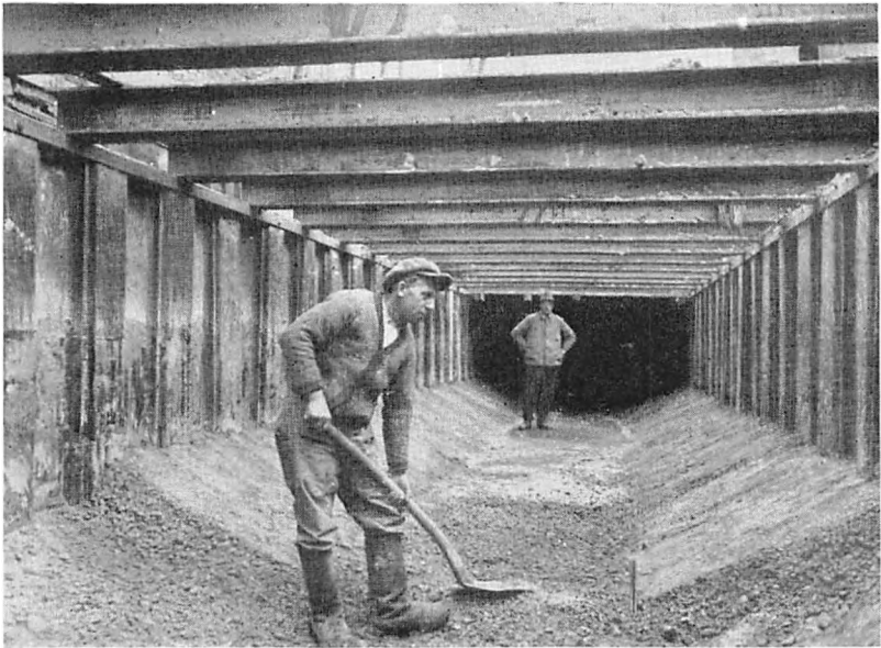
Kildeskovsrenden under Overdækning.
