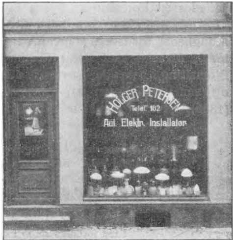
Holger Petersens Installationsforretning.
