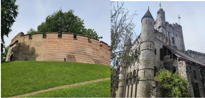
The 'Burcht' castle of Leiden in the Netherlands was built in the 11 th century as a circular wall on top of a hill. Later castles such as the 'Gravensteen' in Ghent, Belgium, were mostly square with towers on each corner
