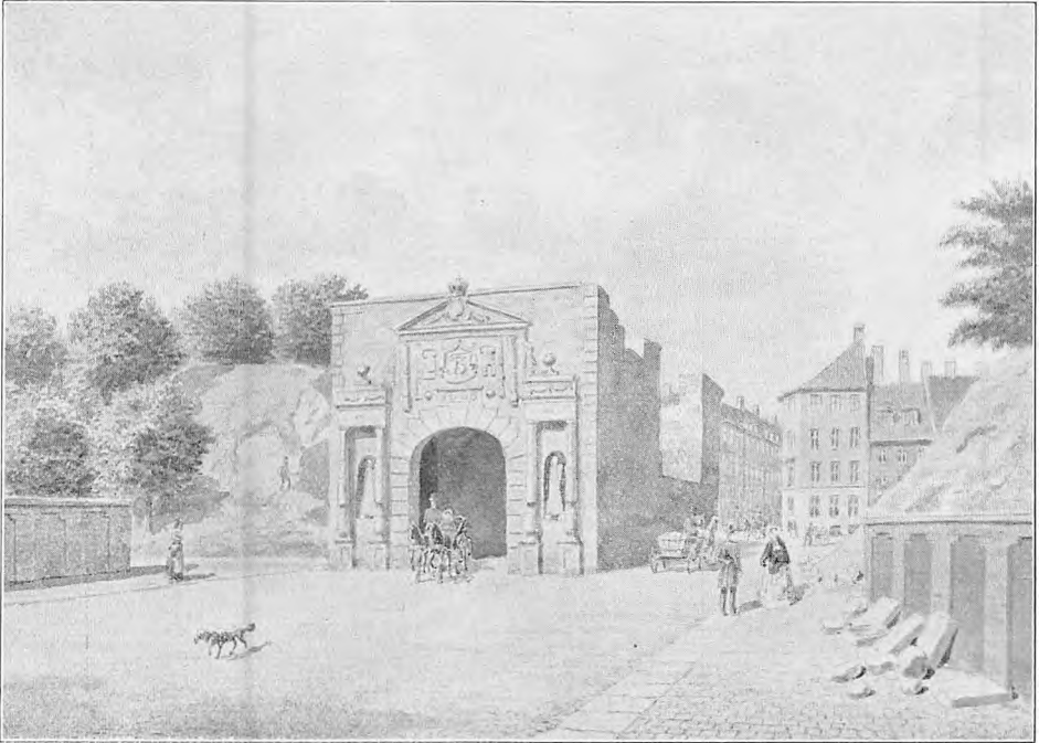
Vesterport under Nedrivning.
