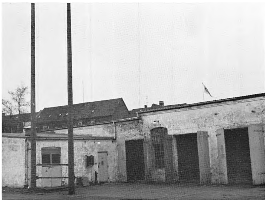
Gl. brandstation i Ringgade.
