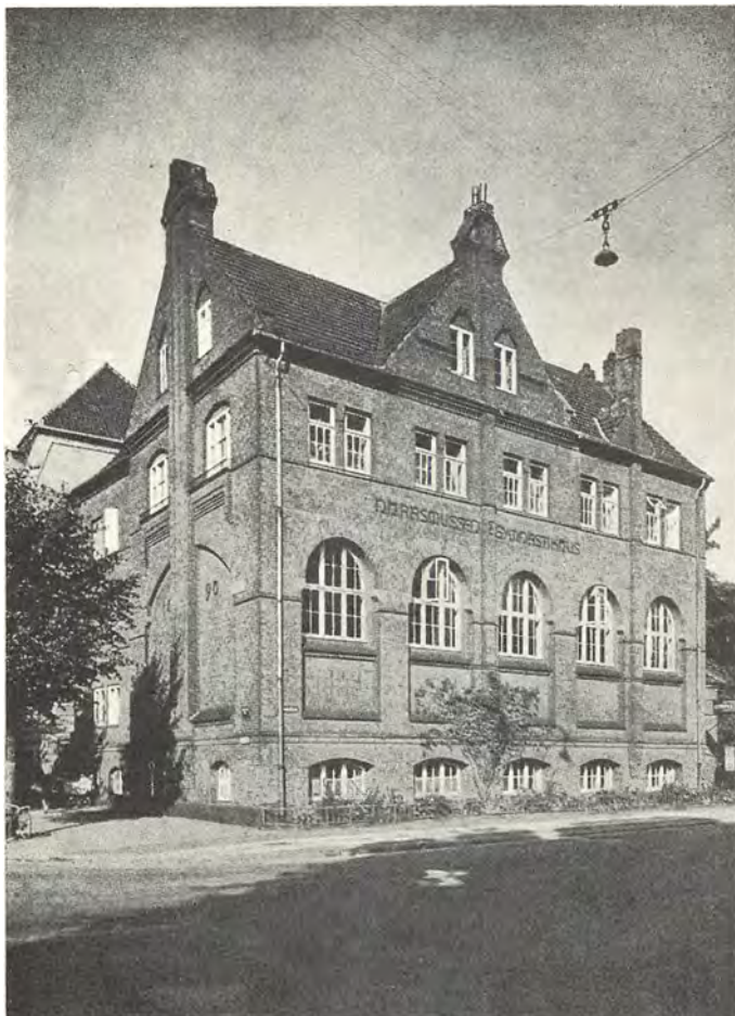
P. V. Jensen Klint: Gymnastikinstituttet, Vodroffsvej 49-51, 1897-98.
