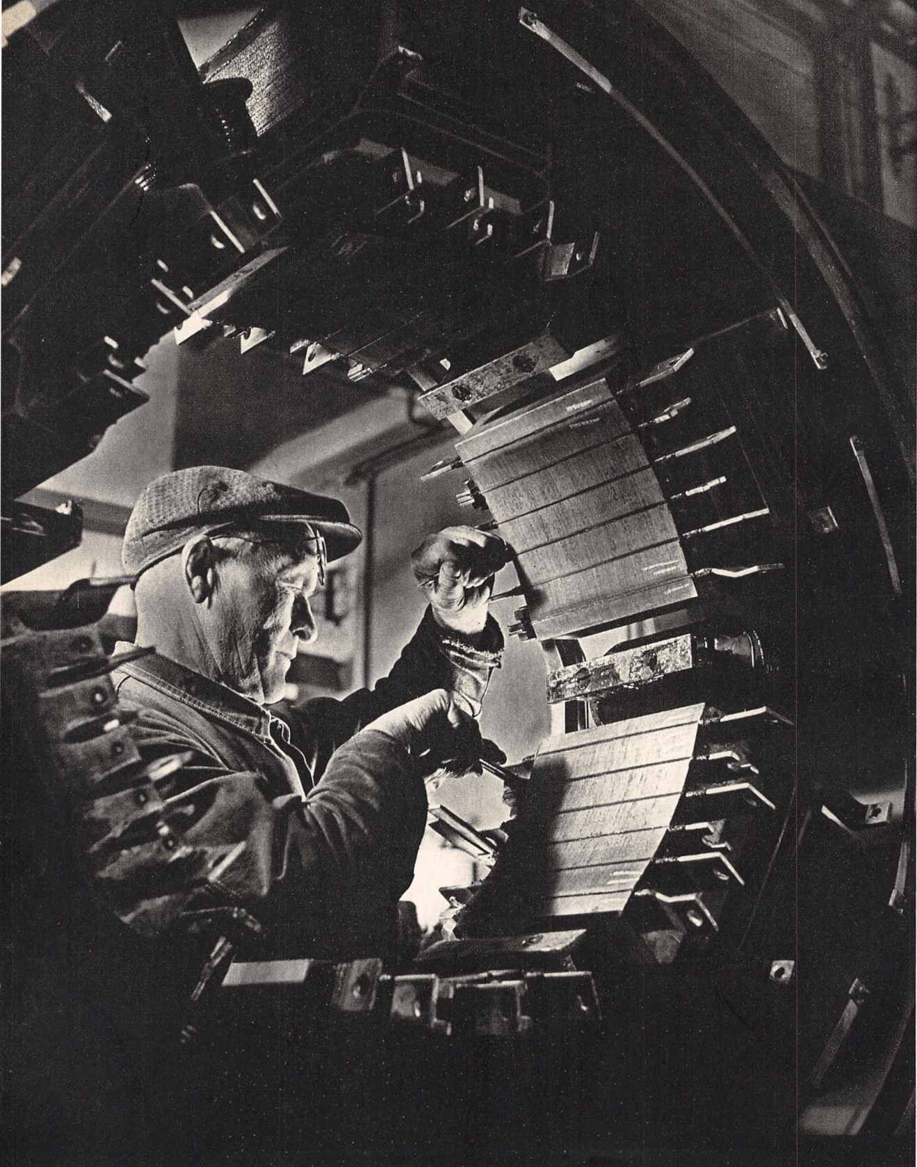
Magnetkran under Montage.
